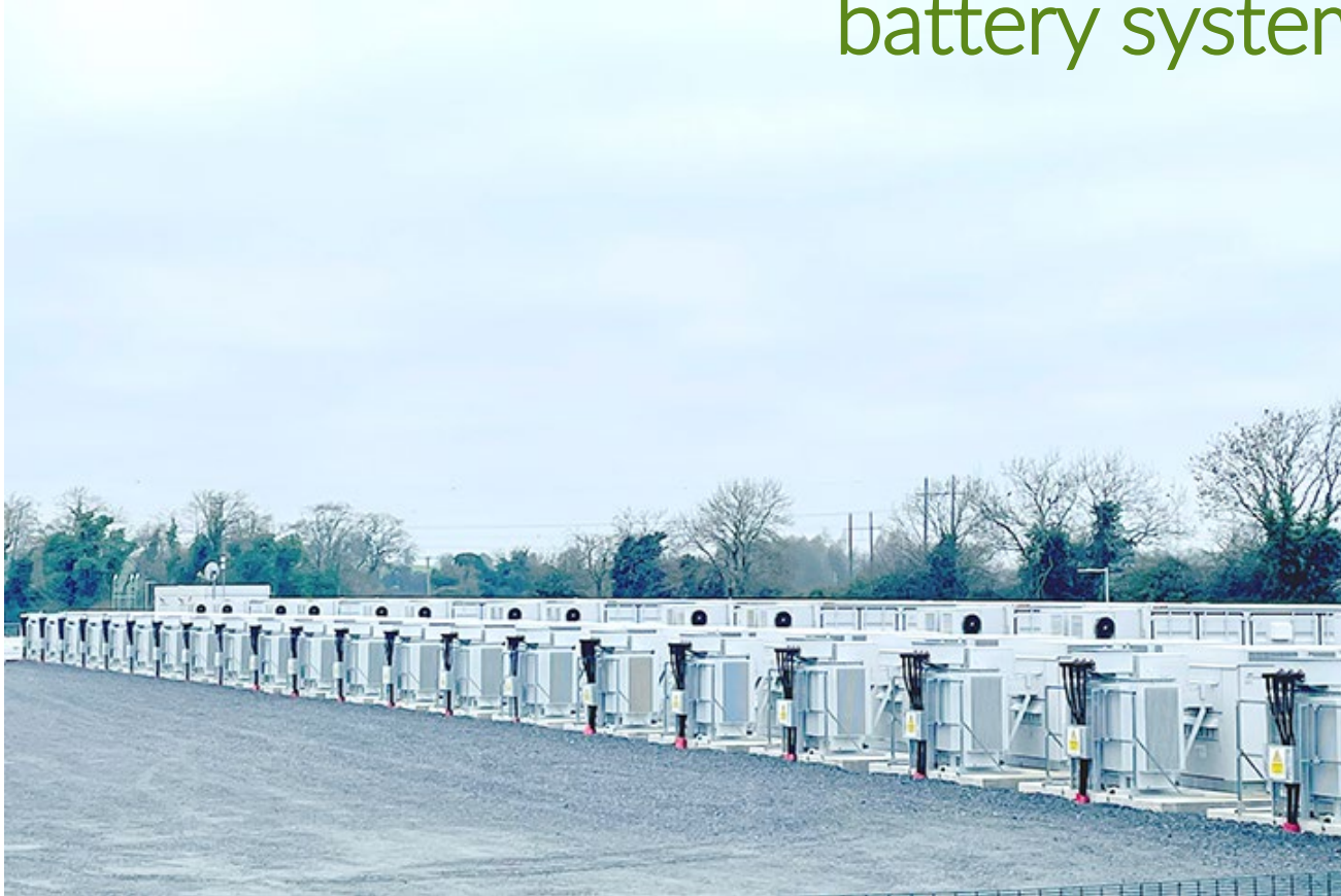
Gorman in Ireland is a 50 MW facility with a storage capacity of 25 MWh
